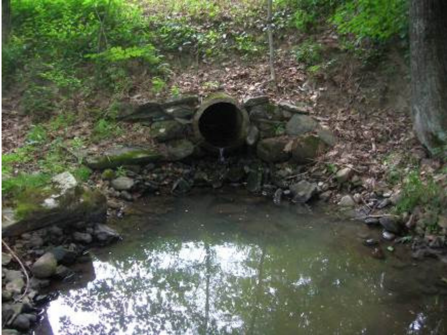
Figure A.24 - Perched culvert above scour pool where brook trout were captured in an unnamed tributary of the lower North River.
