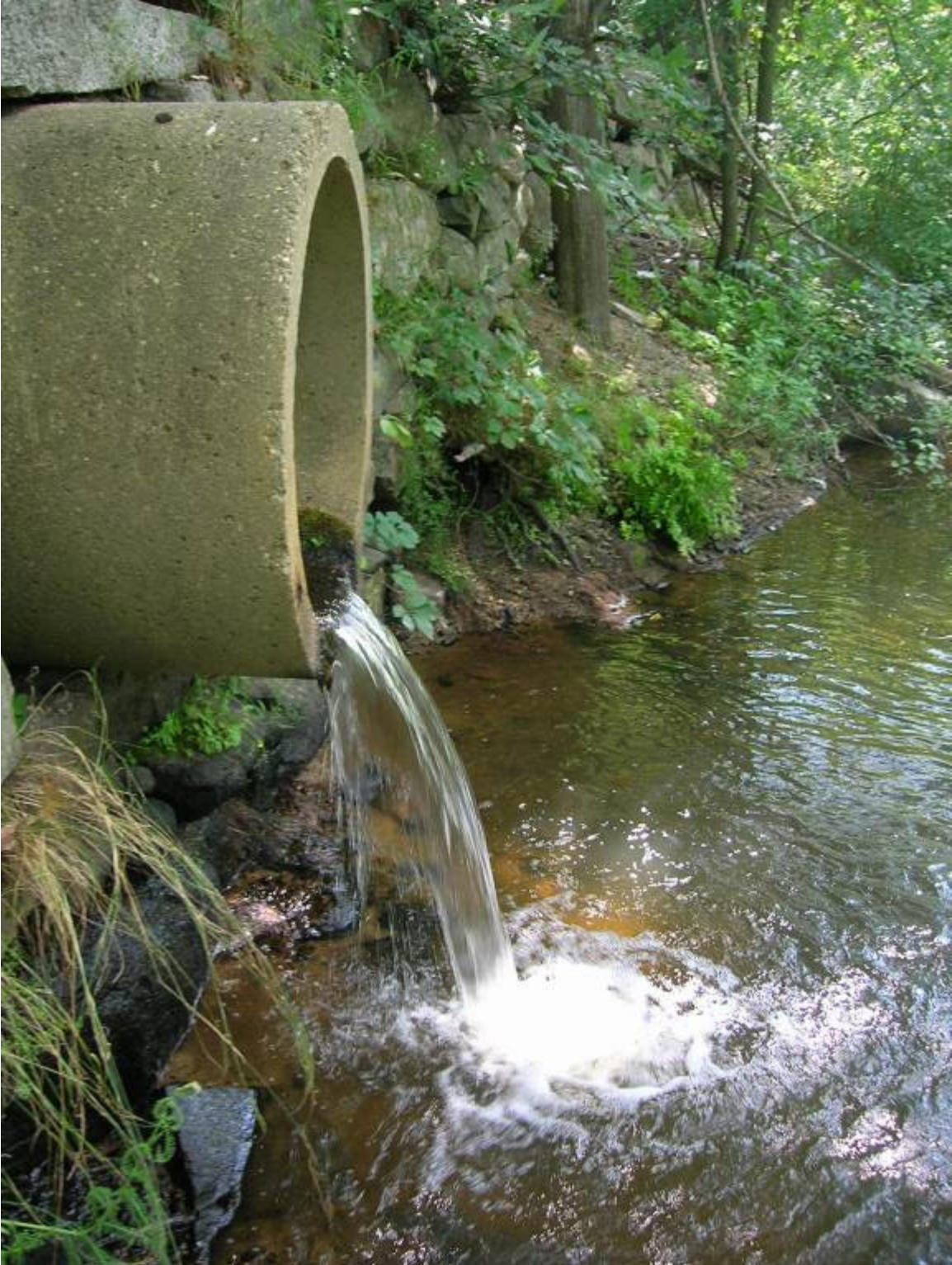
Figure 12. Impassable culvert (perched) on Woodman Brook in the Lower Lamprey River subwatershed.
