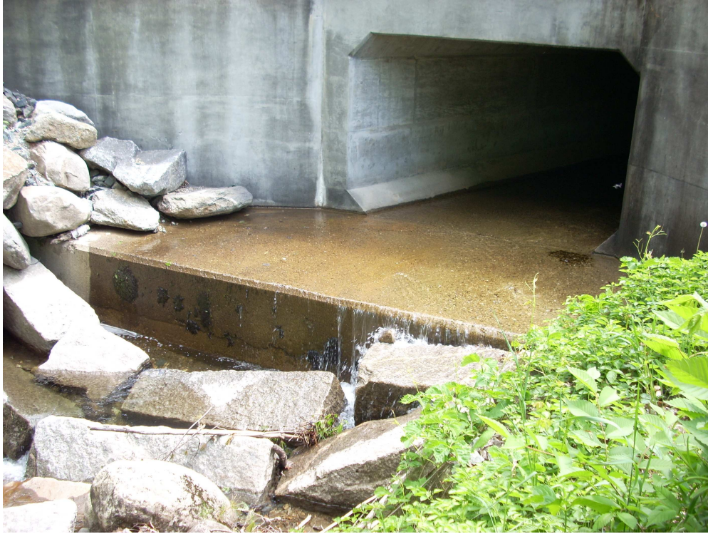
Georges Brook-Hebron. Wild brook trout were found downstream of this culvert and no fish were found for the next 100 meters above the culvert. Road crossing design that does not incorporate fish movement can reduce fish dispersal. Opportunities for fish to repopulate an area or reach more desirable habitat has been reduced.
