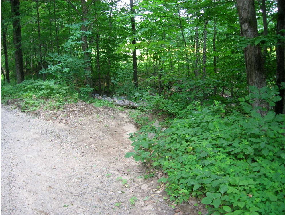
Road design that directs storm water runoff into streams increases erosion and sedimentation rates. This can alter stream habitat and cover spawning substrate, significantly impacting wild brook trout.
