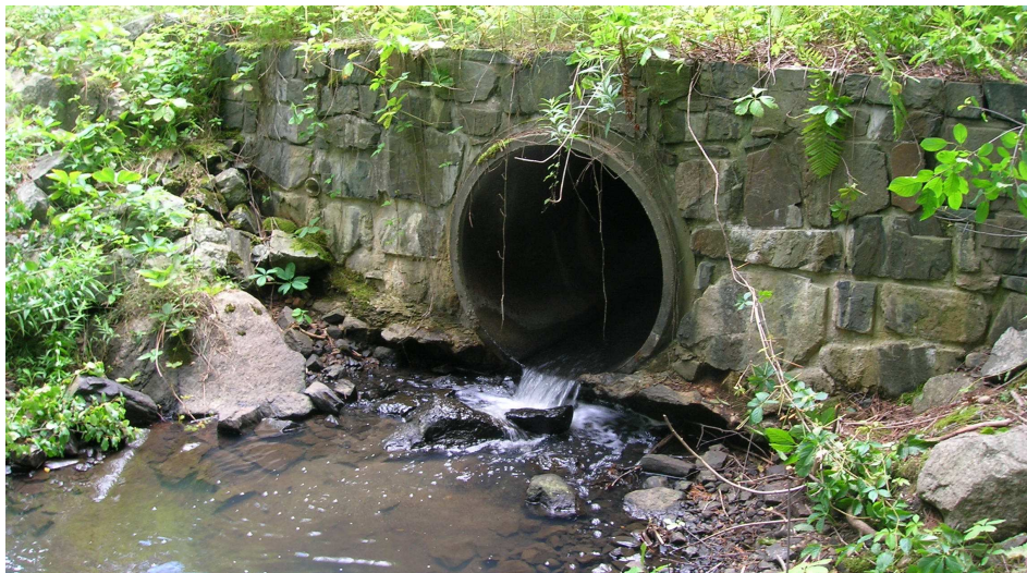
An example of a perched culvert on a tributary to Mink Brook. Crossings not designed with the accommodation of fish passage make it difficult for fish to access more desirable habitats.
