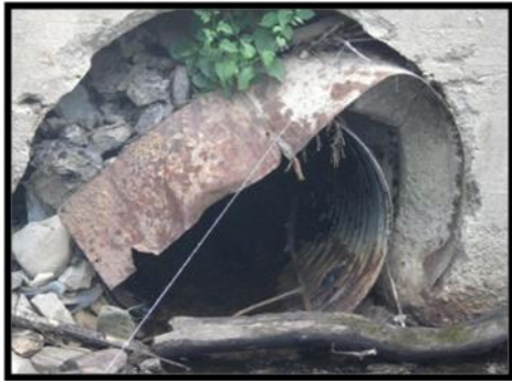
Figure 11. Slip lined crossing on unnamed tributary, Bath, NH.
