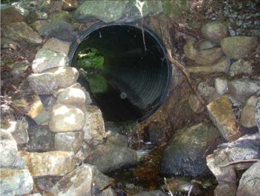
Figure A.6 - One of three Driveway culverts impacting fish passage on a coldwater stream in the Lamprey River Headwaters subwatershed.
