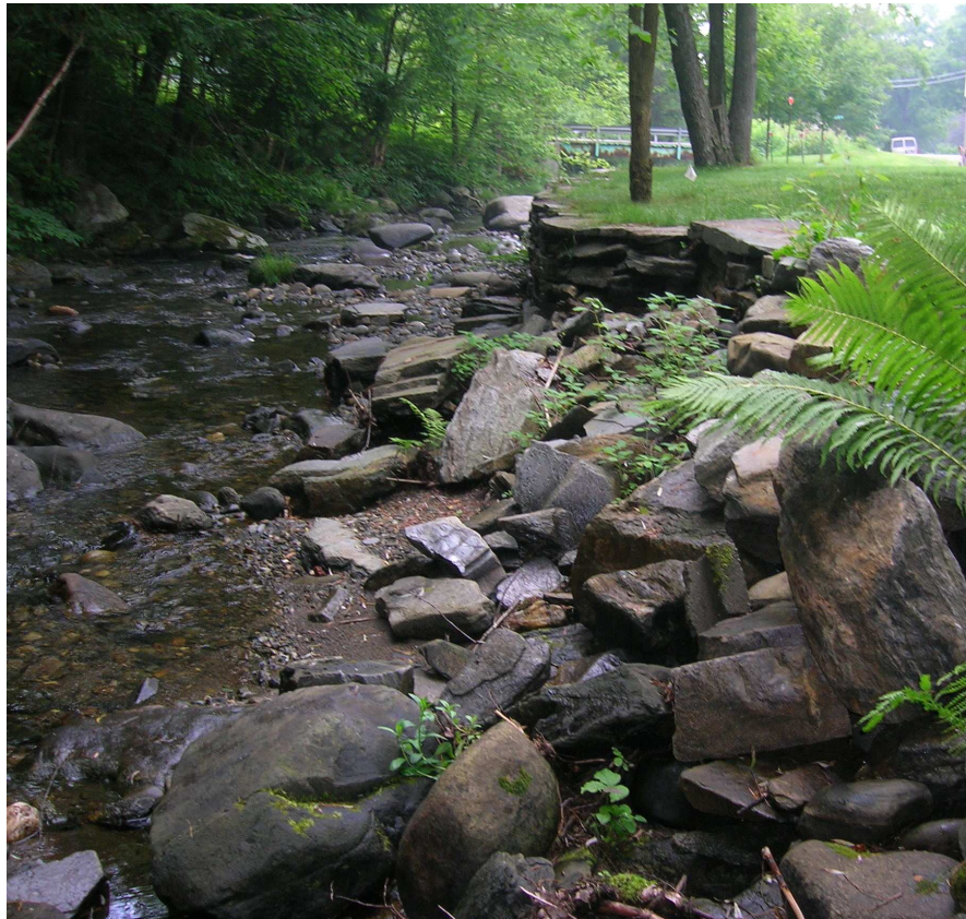
An example of shoreline bank armoring on Mink Brook. During high flows, the stream is precluded from accessing its floodplain where the velocity of flows could be naturally reduced. Instead, erosive flows continue to downstream areas.
