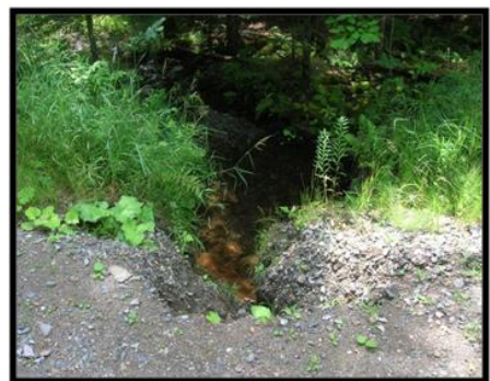
Figure 10. Washout at Unnamed Stream, Bath, NH (site # 14699).
